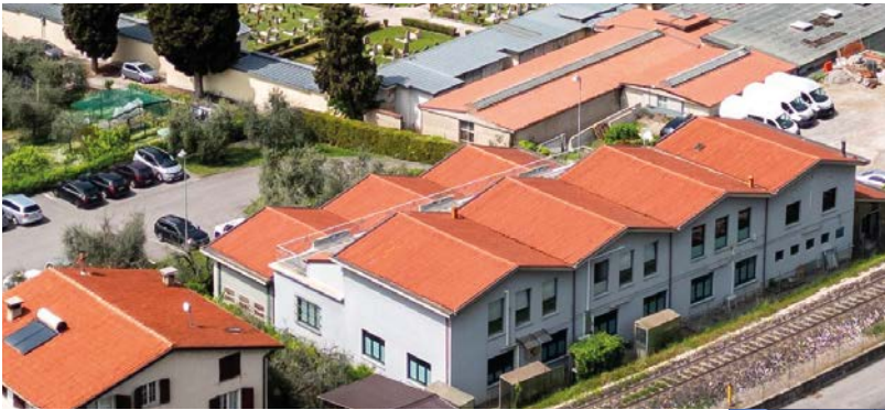
Sale Marasino / Pisogne (Bs - Italy) level, pressure, temperature sensors
